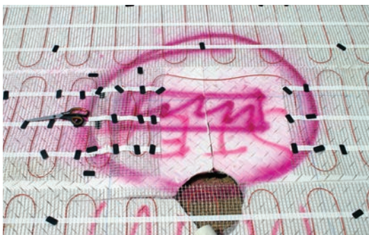
5. Remember to mark goal posts, corner flags, etc. to secure that the heating mat / cables are not damaged when making the holes for the posts.
