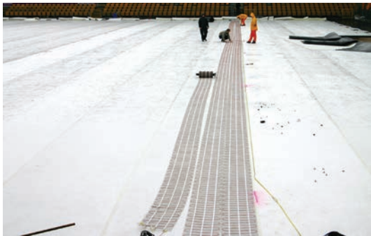
1. Roll out and find the centre of the mat.
