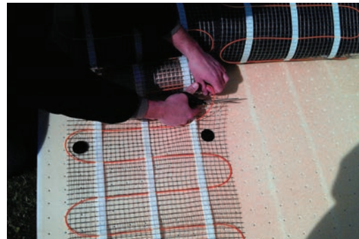
2. At the centre of the mat, cut the mesh - not the cable .
